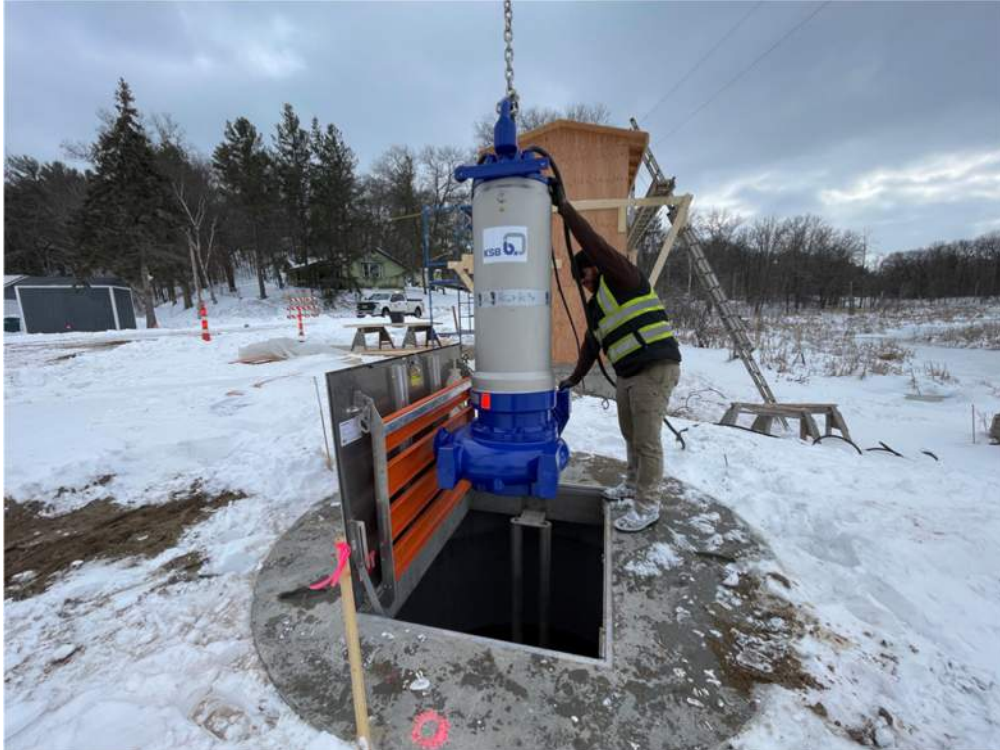
Photo #3: Pump being lowered into the wetwell - Mar 27, 2024, 4:57 PM
