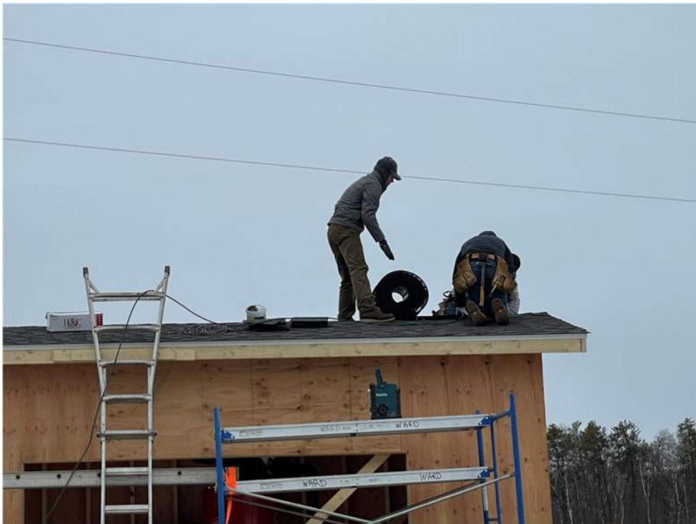
Photo #8: Rolling out and nailing down ridge vent - Mar 29, 2024, 1:51 PM
