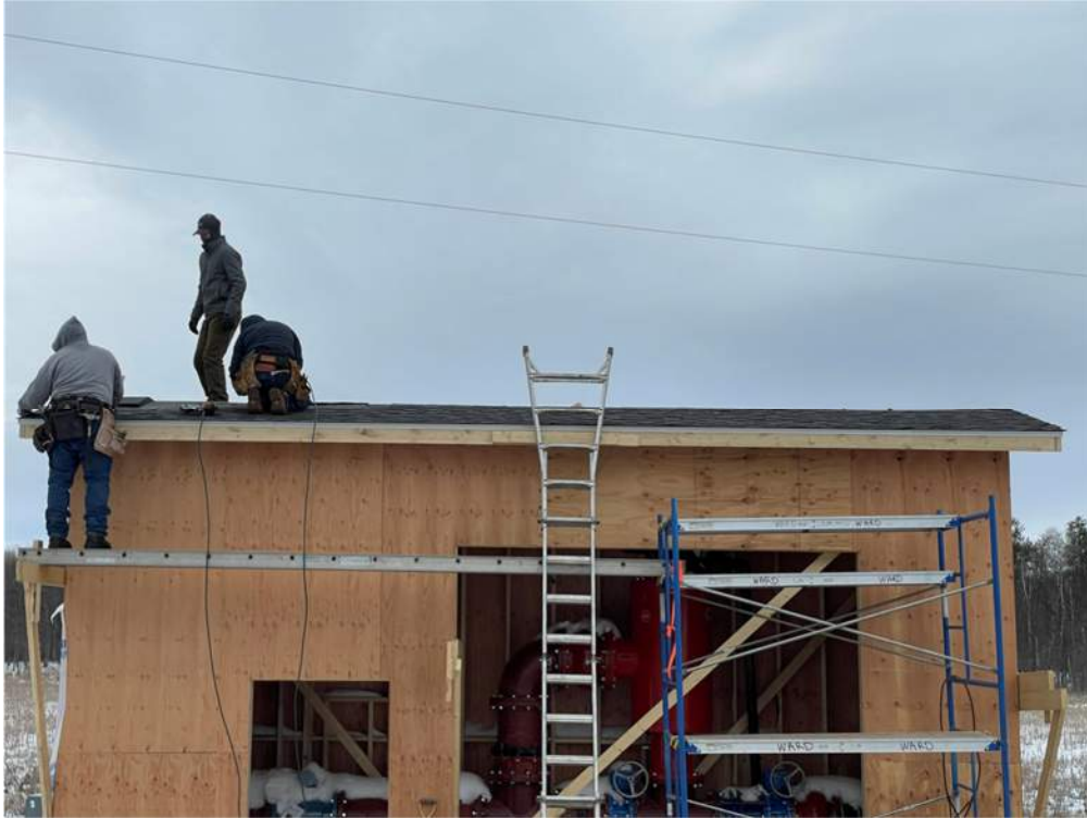
Photo #7: Installing shingles on pump house roof - Mar 29, 2024, 10:10 AM
